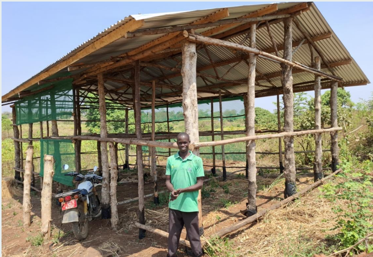
Onencan Kizito in front of his poultry house being constructed
