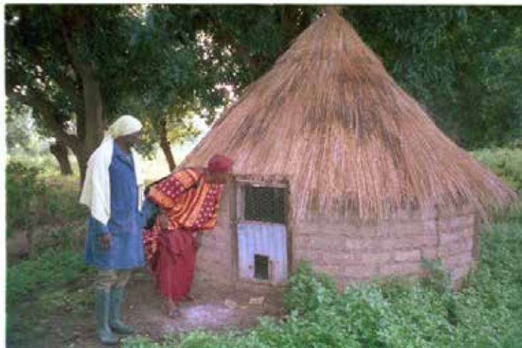
Figure 6: A well-constructed chicken house is placed in the shade, has a high roof and windows with wire mesh, providing good ventilation but preventing entrance of snakes and rats. The door is facing south or north to avoid direct sun. The door is big enough for a person to enter to clean the house frequently (source Riise et al 2004)
