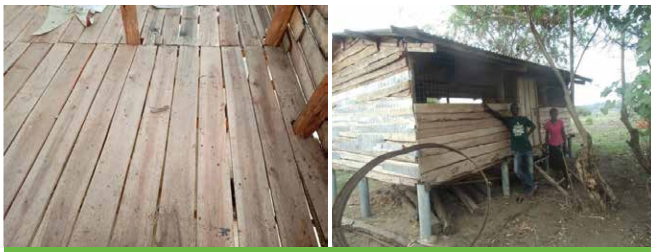
Figure 7: Raised house with slates built by youth in Pakwach. The inside has timber with spaces in between to allow removal of the droppings.
